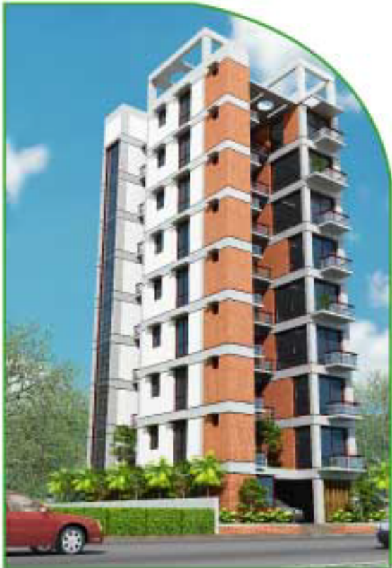
Vista HS Tower @ Aftabnagar
