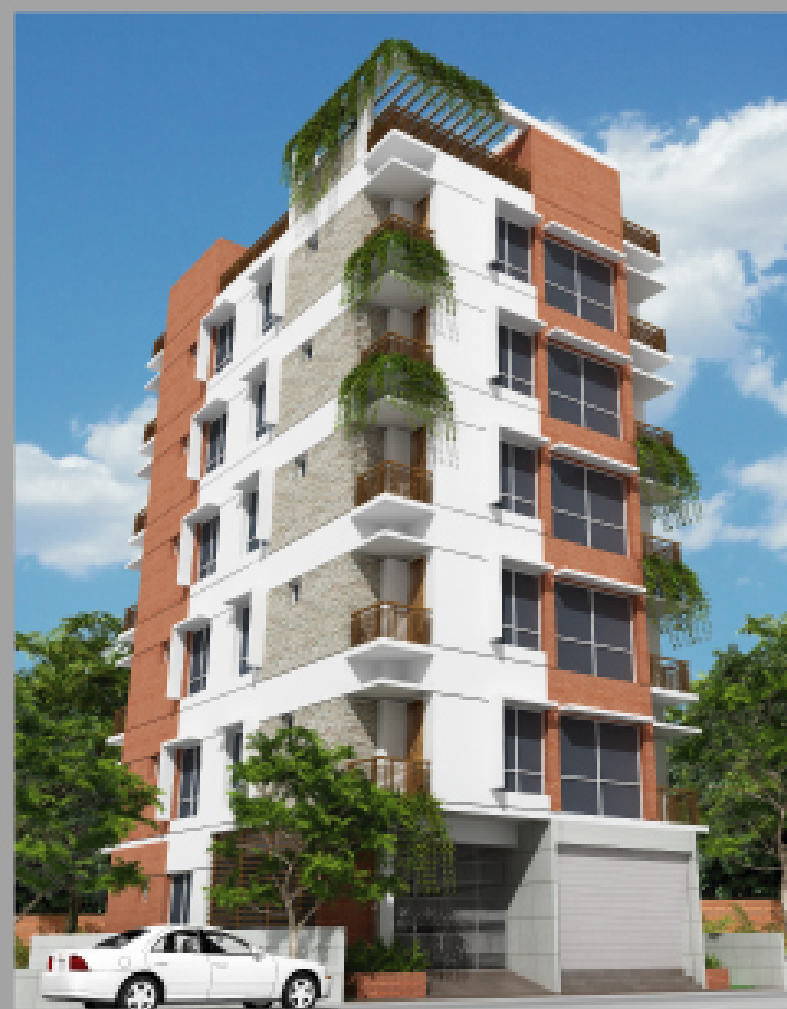
Up coming Project @ Mirpur-11, Dhaka.
