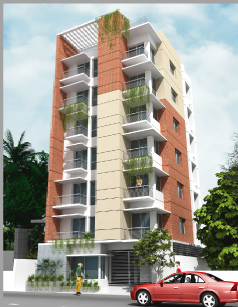
On going Project @ Mirpur-2, Dhaka.
